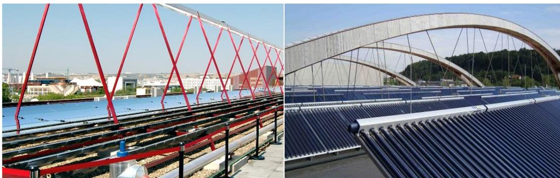
Left: Fresnel-collector. Right: Plant with evacuated tube collectors: Industrial Solar and Ritter XL Solar can offer their customers now solar thermal installations for industrial applications within a temperature range of 60 - 400 °C.
